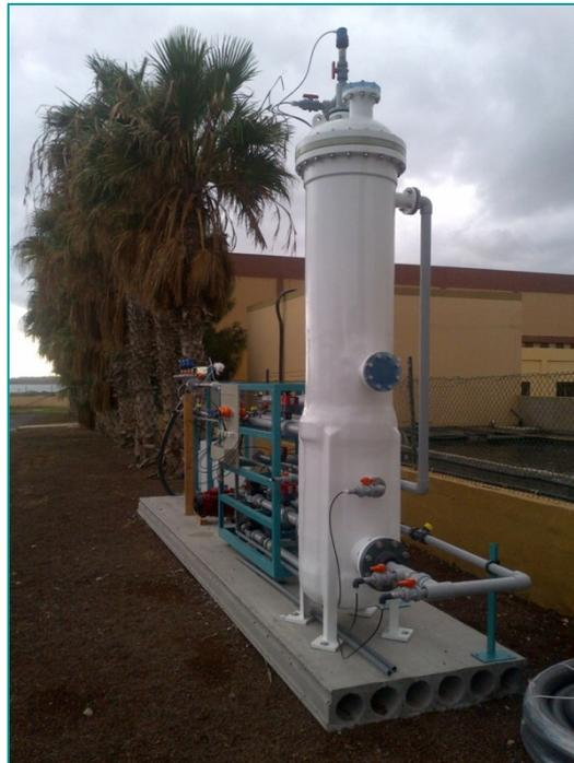
Figure 2: Pilot i-UF400 installed in Southeast Supramunicipal District waste water Treatment Plant, in the municipality of Agüimes on the island of Grand Canary; Spain
